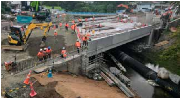
The new Walmsley Rd Bridge under construction over Te Ararata Creek.
