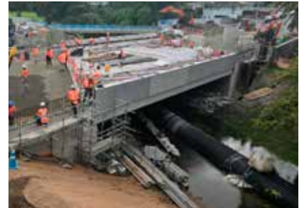
Construction of the Walmsly Road bridge.
