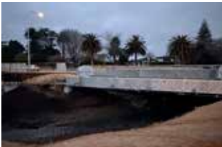
The completed bridge over Te Ararata Creek.
